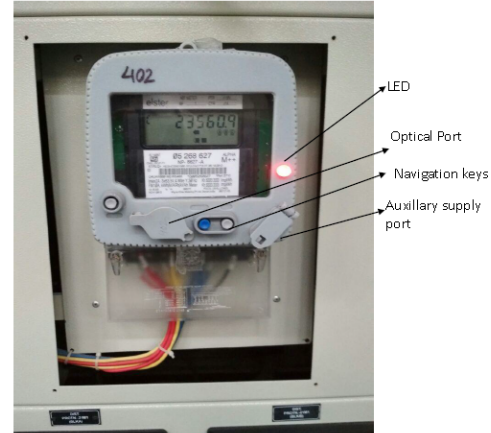
Main meter: NP-8627 A Model- Alpha A1640
