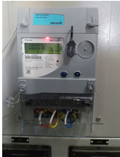
Main Meter – NP 2985A (Secure) Model E2M021
