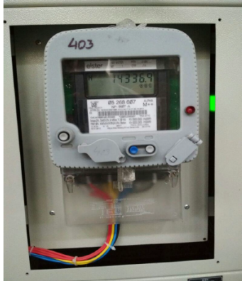
Main meter: NP-8607 A (Elster) Model- Alpha M++
